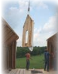
The roof is hoisted and end panels are added.
