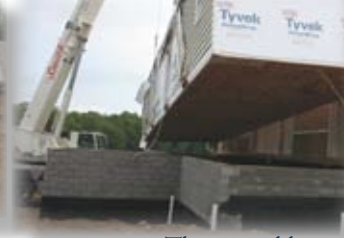
The second box is hoisted into place and the crew makes sure that it is set tightly against the first box. The boxes are placed in order until all five boxes are in place.
