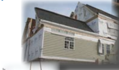
Top flips are assembled and sheathed on the ground and craned into place.
