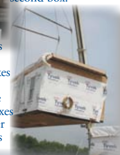
With one box in place it is time to hoist the second box.
