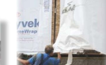
As the second box is set, the third box is pulled in to be prepared for its lift.
