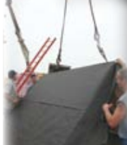
Top flips are assembled and sheathed on the ground and craned into place.
