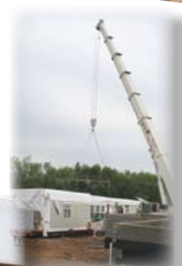
With one box in place it is time to hoist the second box.
