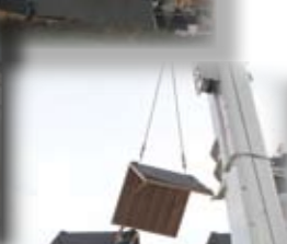
As the second box is set, the third box is pulled in to be prepared for its lift.
