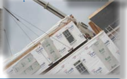
The second box is hoisted into place and the crew makes sure that it is set tightly against the first box. The boxes are placed in order until all five boxes are in place.
