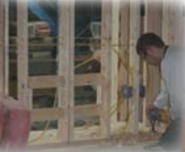
Walls are built, lifted into place, and fastened to the floor.
