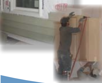
Electric is run and the insulation is installed. The home is sheathed, wrapped with Tyvek, then the windows and siding are installed.
